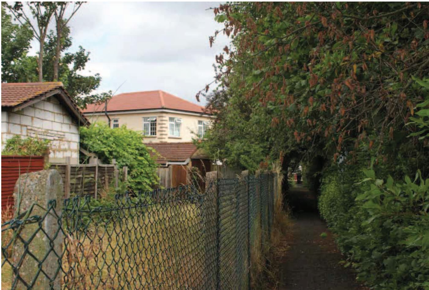
Figure 6: Block of flats on land to the rear of 125 Kenley Road
