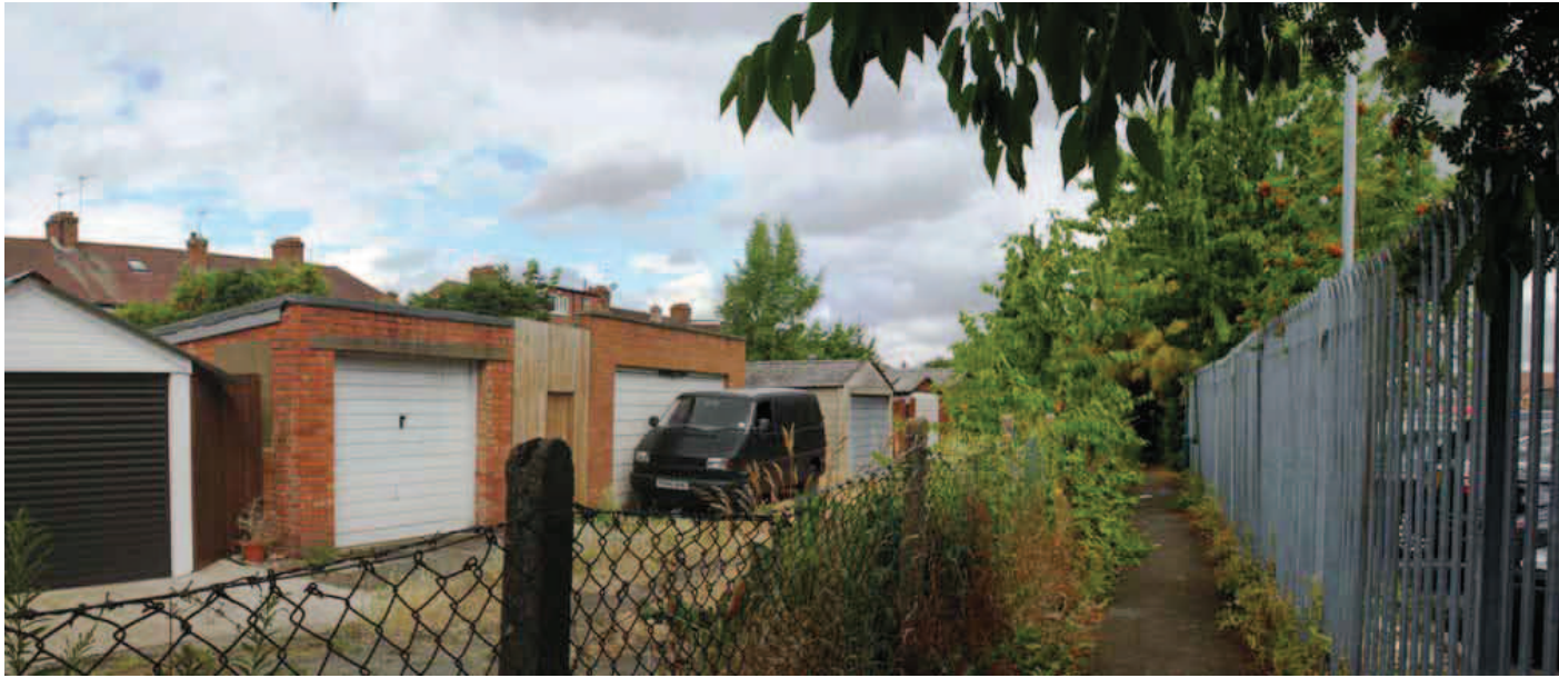
Figure 5: Public footpath garages at the rear of houses facing onto Windermere Avenue
