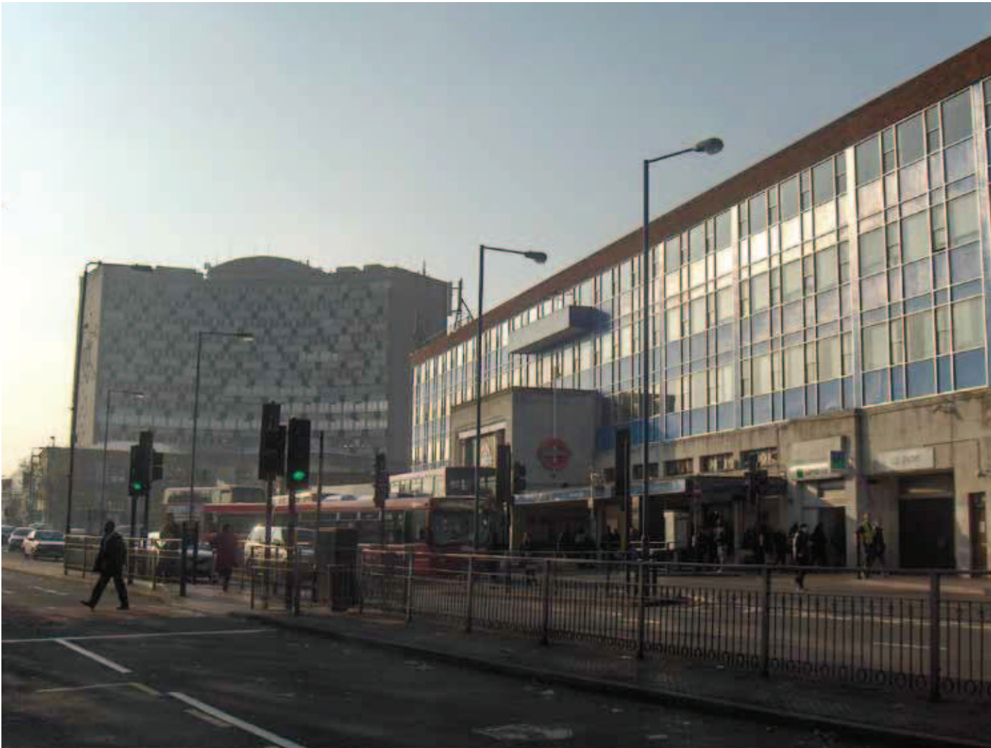
Figure 14: Public realm in front of station requires improvement
